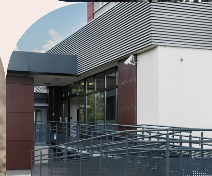
Removal of architectural barriers
